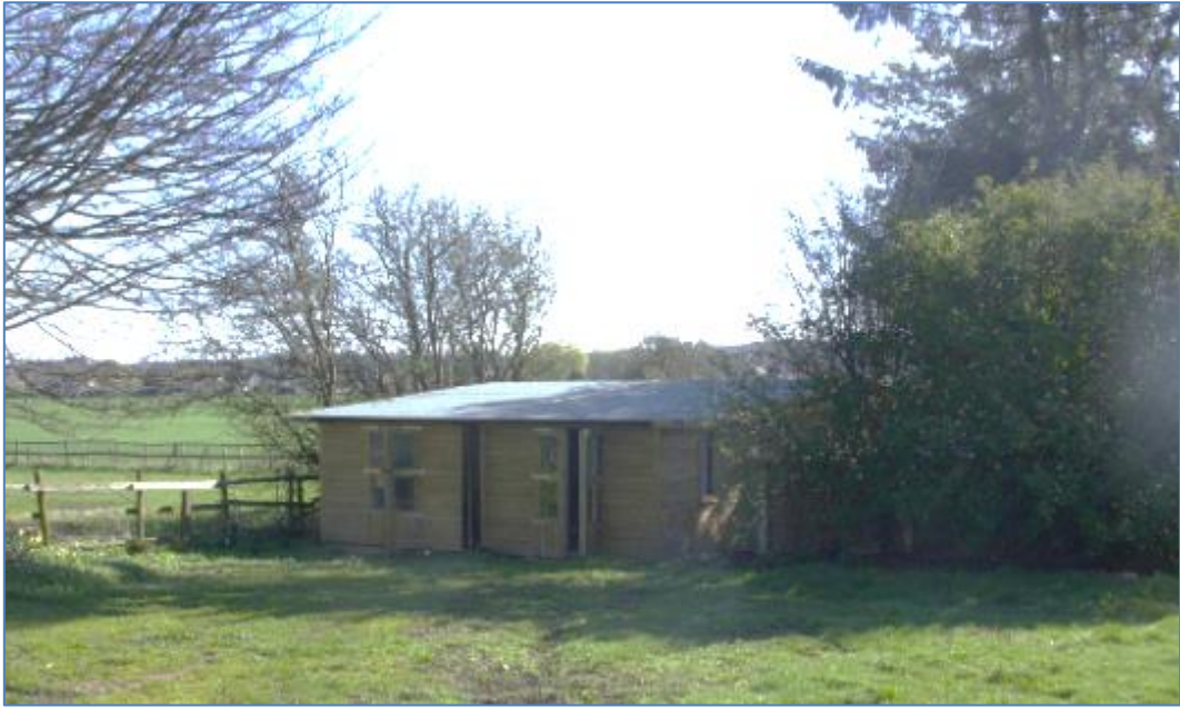
Unauthorised buildings on the land.
